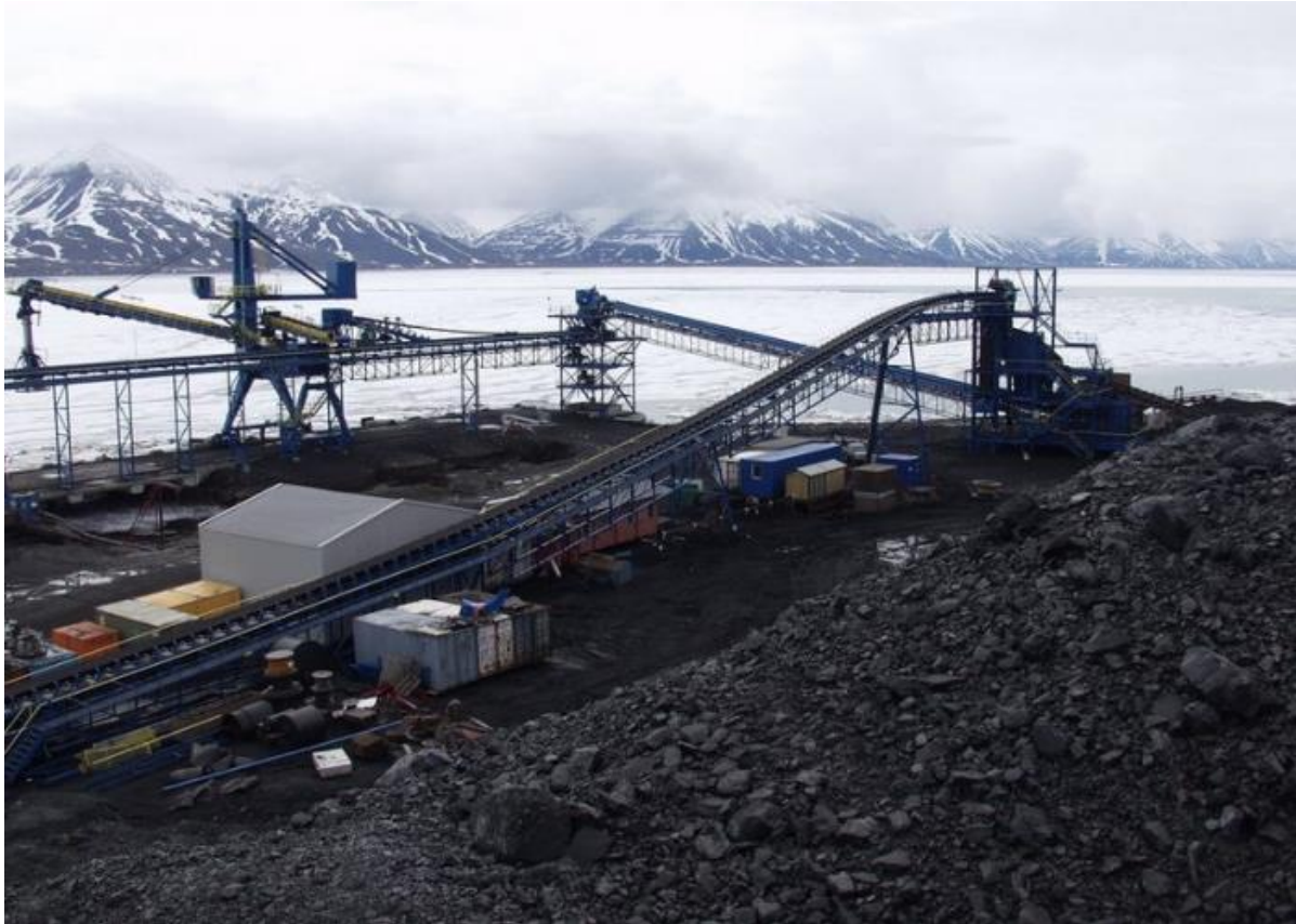
Coalharbor from where the Svea coal is shipped to the world markets. Photo: Thomas Nilsen / BarentsObserver
